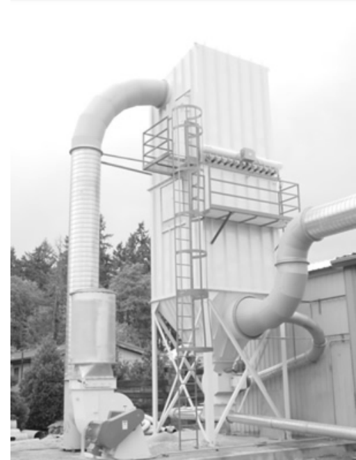
Bag house batch treatment concept
